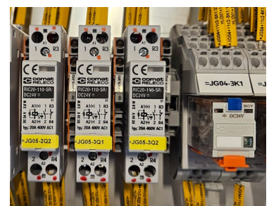
RIC railway contactor for controlling motor control relays in various applications
