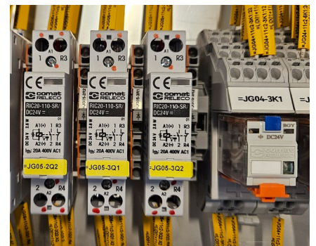
RIC railway contactor for controlling motor control relays in various application
